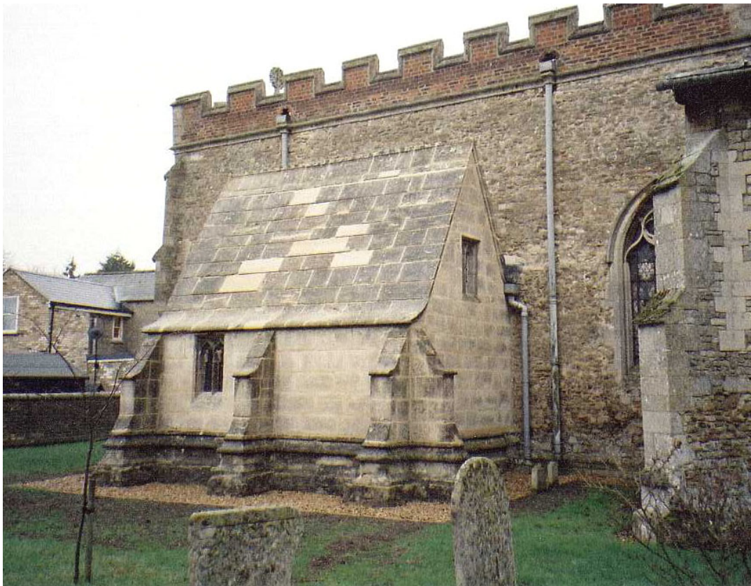
...and after work was completed.
