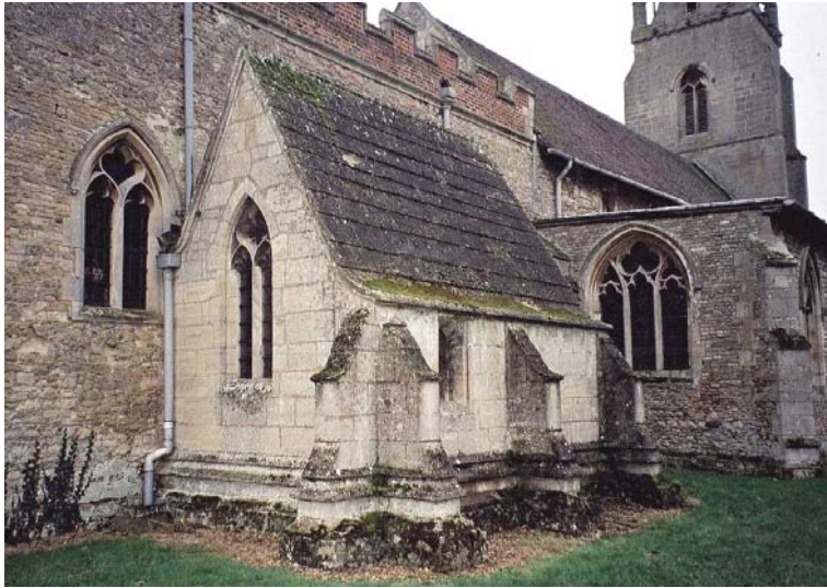
The Sacristy prior to conservation work...
