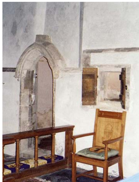
The squint door and niche from the chancel (note blocked chancel window above door)
