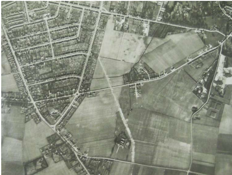
The tank trap is visible as a white scar running north south across what was then open fields either side of Queen Ediths Way (Addenbrookes would eventually occupy the land bottom left of photo)
